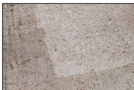
ROUGHENING CONCRETE
